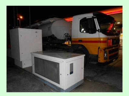
The VR Refiner is an advanced system that processes displaced petrol vapours at the Fuelling station during product transfer and converts it to re-saleable fuel.
