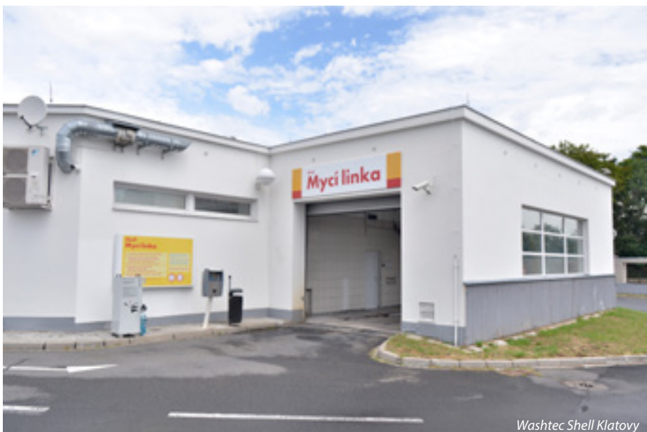
Washtec Shell Klatovy
